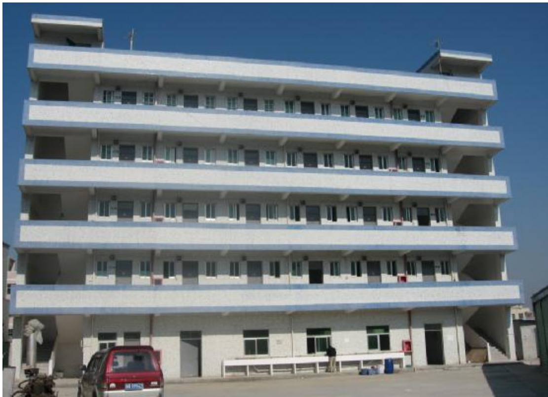
Metal work section
